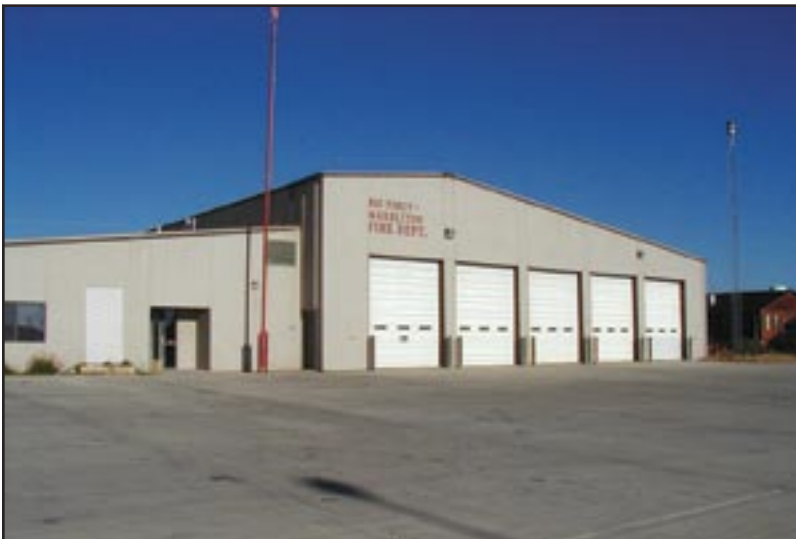
Big Piney/Marbleton Fire Hall. PINEDALE ONLINE PHOTO
