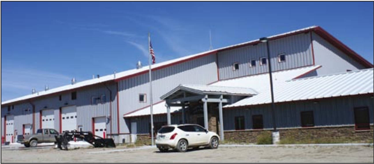
The County Road and Bridge shop near Pinedale.
